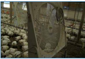
In addition to circulation fans, some open-sided houses are also equipped with spray nozzles (foggers) that lower the house temperature through evaporative cooling.
