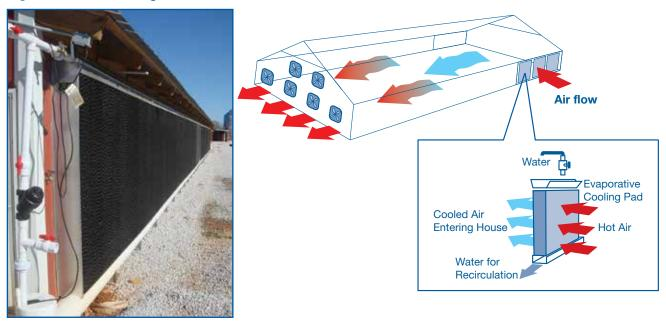
This design and layout of the cooling pads allow the large volumes of air used in tunnel ventilation to enter through the pad surface area and be cooled before entering the house.
