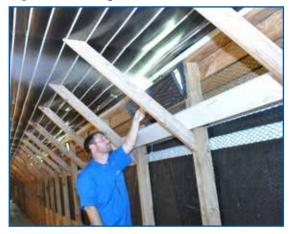
When smoke testing a house, it is advisable to do it under "worst case" conditions. That is, when the house is at brooding temperature and the ambient temperature is at, or close to, as cold as it may get.
