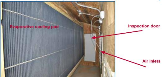
For the tunnel ventilation system to operate efficiently, it is important that the cooling pad area is properly calculated based on the total operating capacity of the fans.
